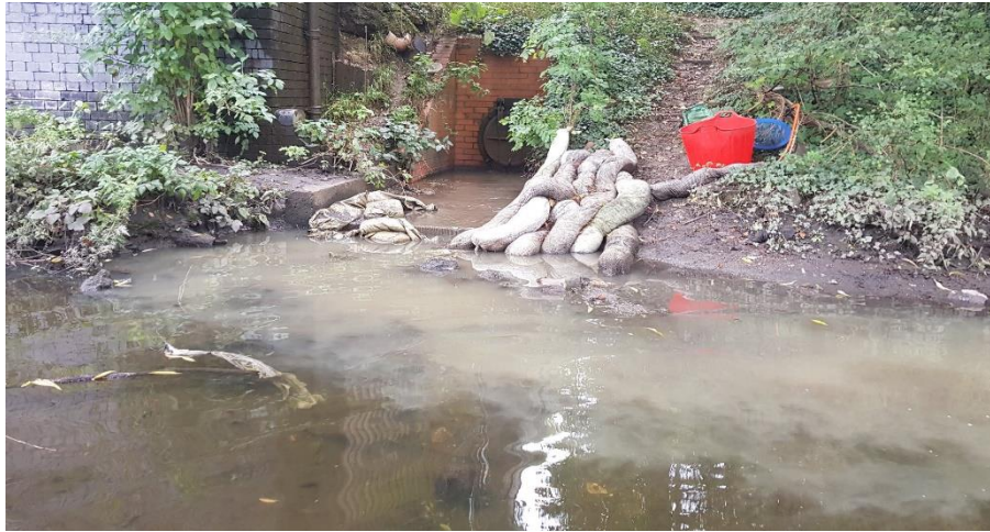
Figure 14 - Discoloured water flowing from Oxhey Park outfall. Source: CCP CIC
